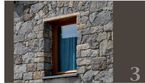
Window architrave with support strip
