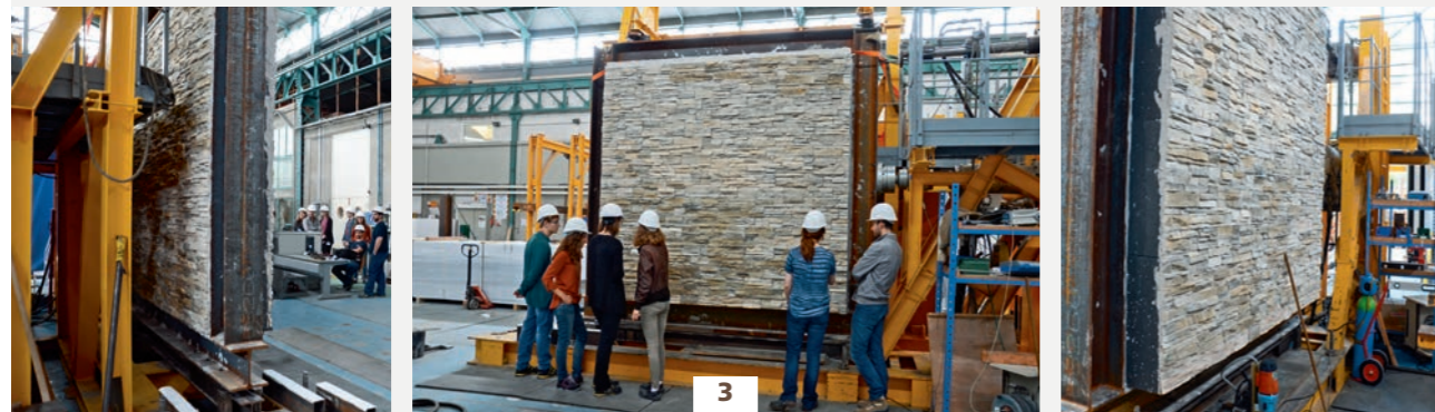
muregeopietra on concrete blocks
